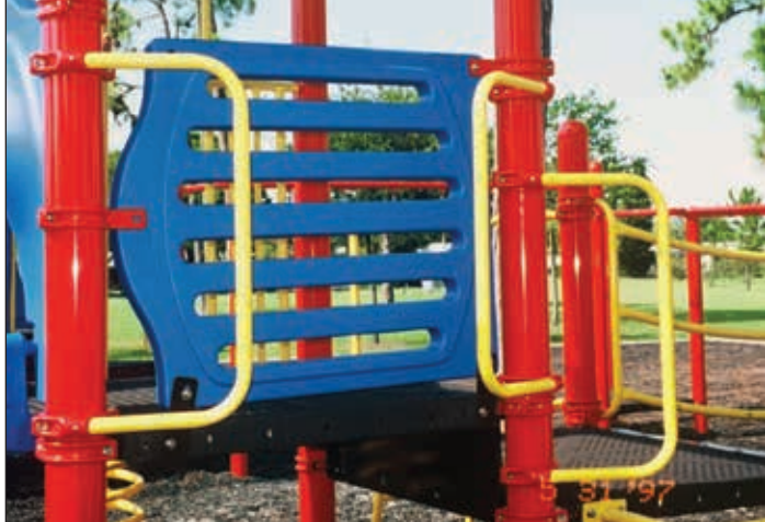
THIS "REPAIR" JOB TO A BARRIER WALL CREATED A CLIMBING HAZARD — Photograph by the Author
