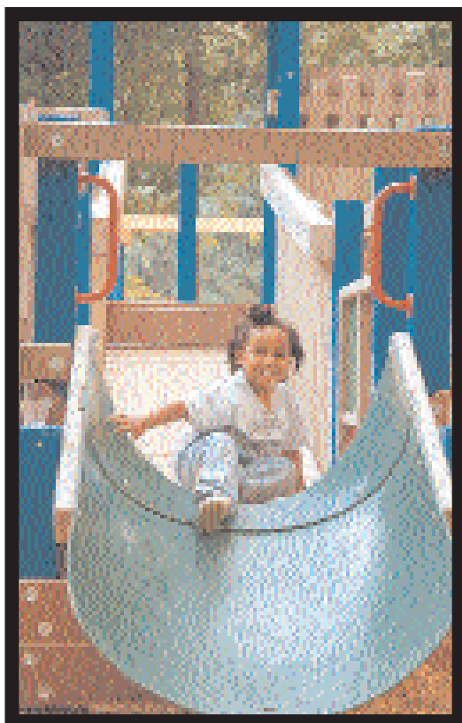
Photo by author. Children in wheelchairs are able to access this slide. There is a transfer platform behind the slide so children can move from a wheelchair and use the slide. The WOODCARPET™ used in the fall zone around the slide is wheelchair accessible.
